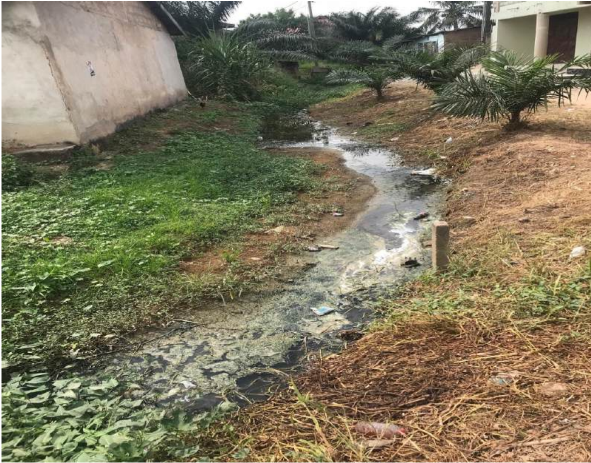
Fig. 4.2b: A photo of the recent state of ditches in the community with sand almost filled to the brim.
