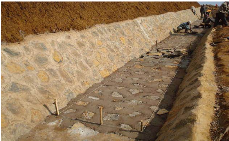
Fig. 5.1: A stone-pitch under construction.
