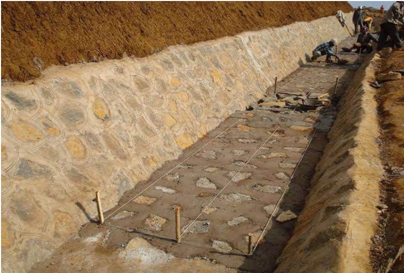
Fig. 2.2b: A stone-pitch drainage under construction .
