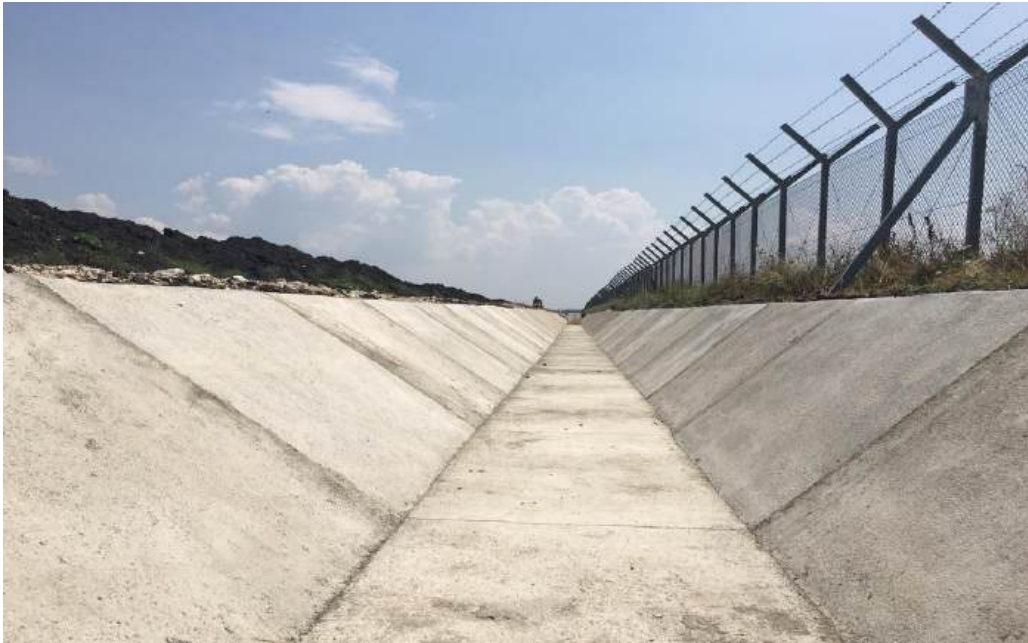
Fig. 2.2c: A 3.5km open v-ditch drainage channel.
