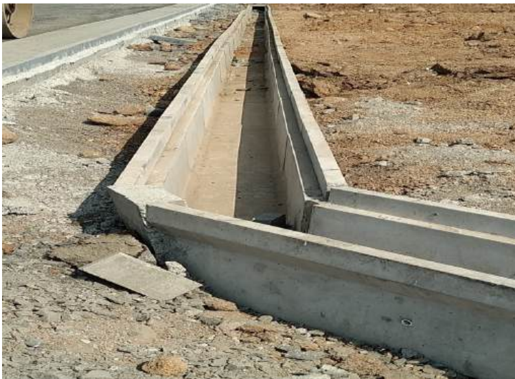
Fig. 2.2a: A roadside u-drain.
