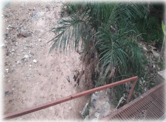
Figure 4.2.4: Broken bridge railings
